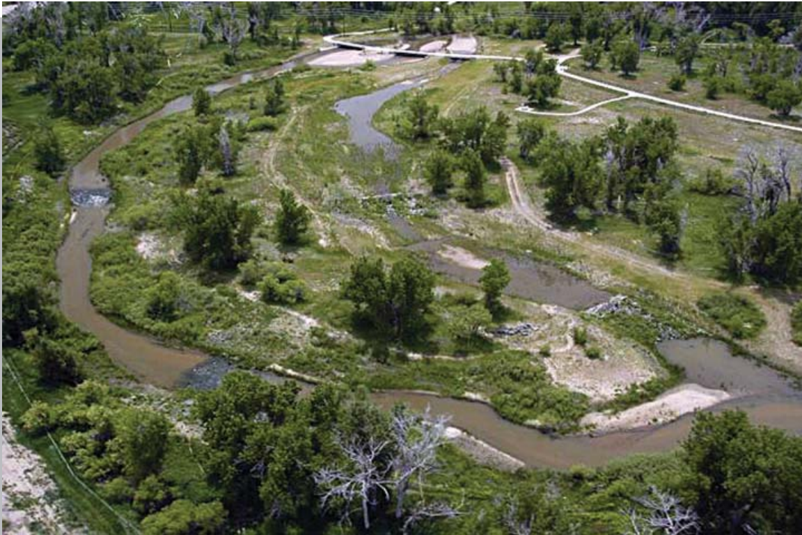
Figure 4 - Aerial photo of Cherry Creek at 17-Mile House stream restoration project. The project included the creation of a new secondary channel to distribute surface water. (Photo courtesy of Muller Engineering Company).
