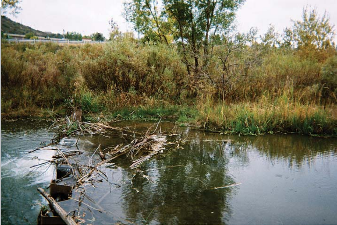
Figure 3 - Example of sheet pile cutoff drop structure on East Plum Creek in Castle Rock, Colorado used to enhance Preble's habitat.
