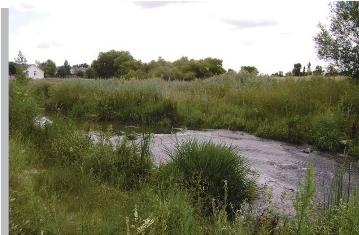
Figure 5 - Cherry Creek at Stroh Ranch stream restoration project. Looking upstream at small riffle structure. Wetlands have expanded upstream of the structure.
