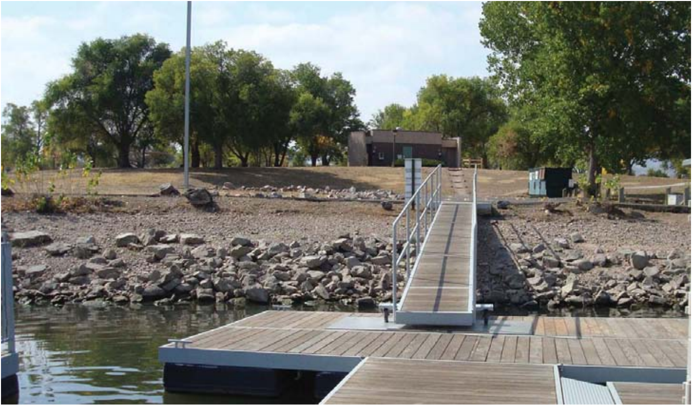
3-15 Fuel Dock Gangway
