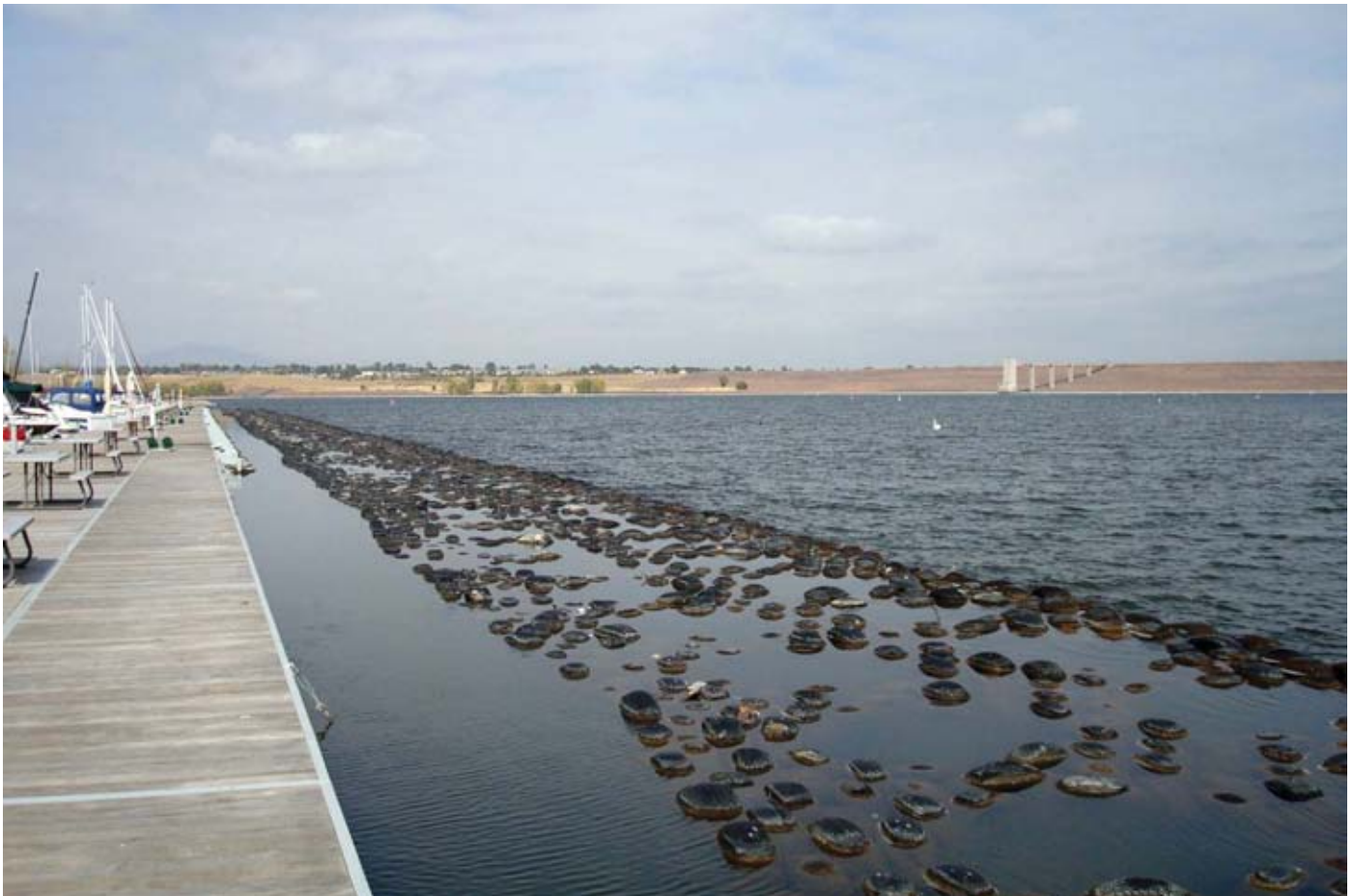
3-5 Floating Tire Breakwater
