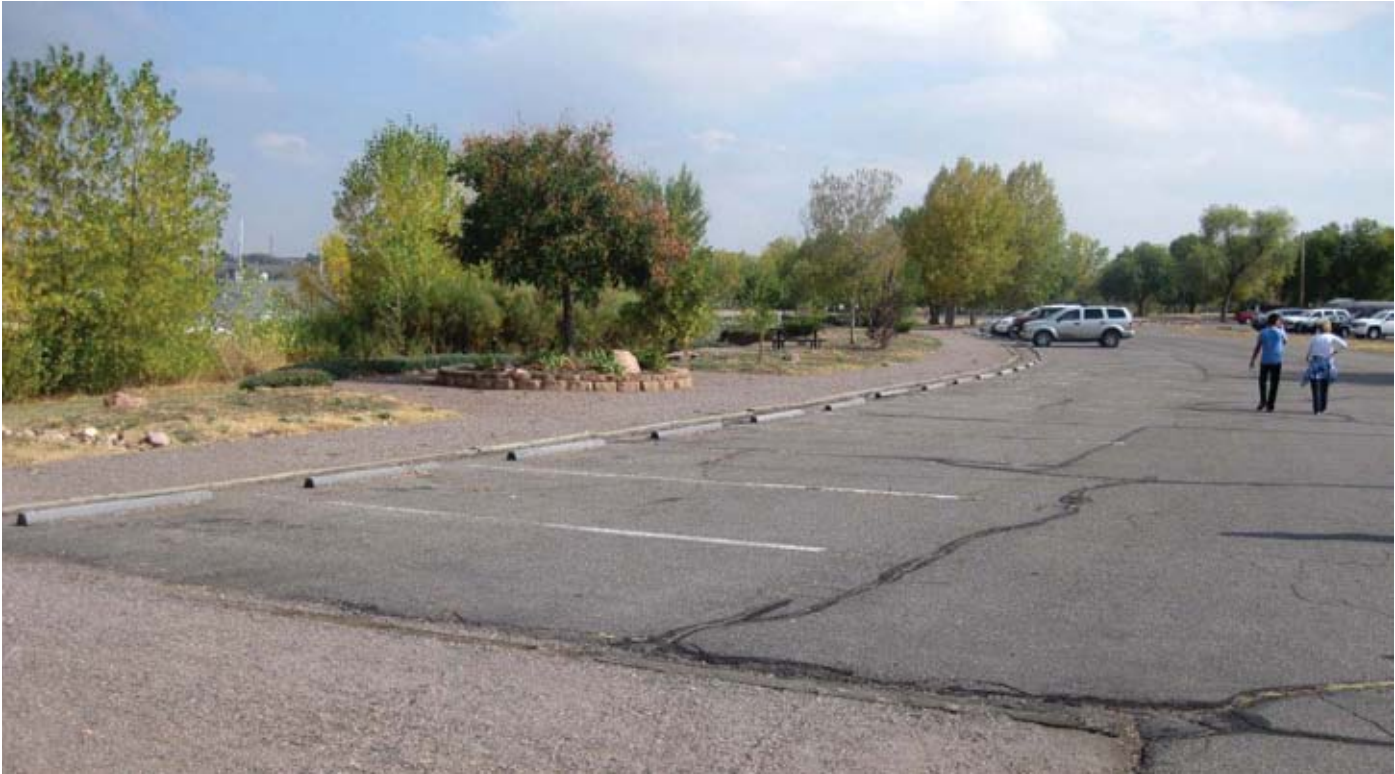
3-17 Existing Parking Lot
