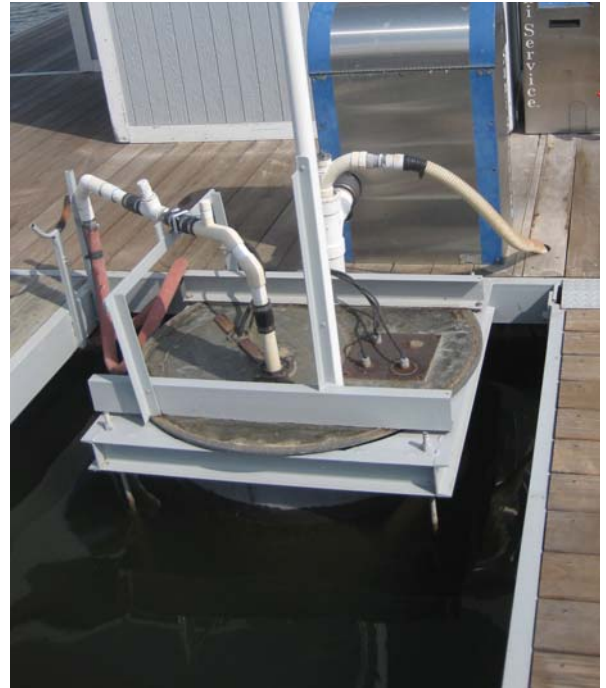
3-11 Pump Out Station
